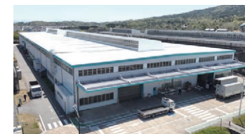
Heat-shielding measures at plants (heat-shielding coating applied to roofs and wall surfaces)
