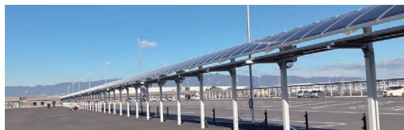
Film-type perovskite solar cell bus stop shelter
