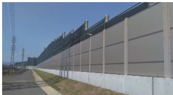
Soundproof privacy walls incorporating acoustic control technology into an exterior product for plants and other facilities
