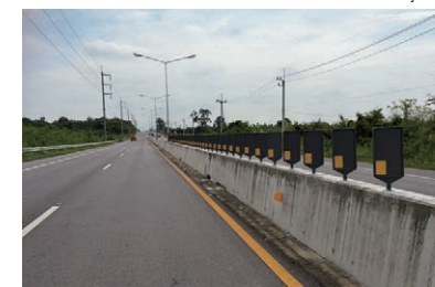
Project for anti-glare panel installation on national highways in Thailand
