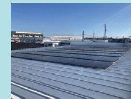
Solar panels installed on the roof of the admin/welfare building
